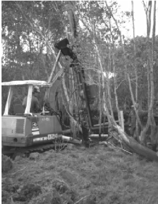
Fig 8. Driving Piles in mangroves
