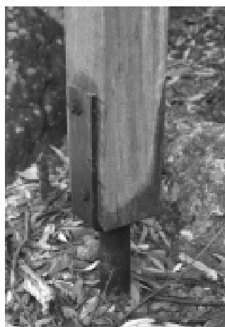
Fig 10 Rock baseplate in cored hole
